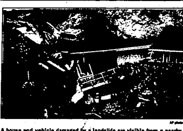
A house and vehicle damaged by a landslide are visible from a nearby hilltop Wednesday in Laguna Beach, Calif.
