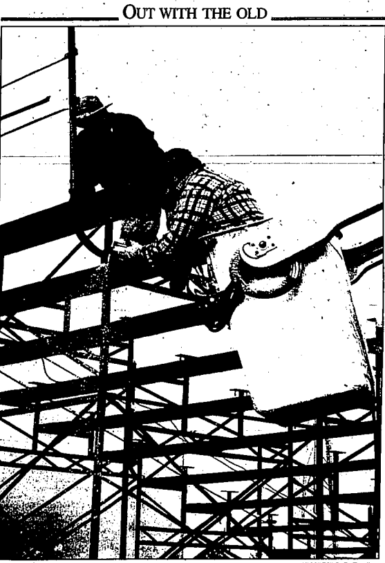
School district employees Max Brown and Steve Bennet, right, use a cutting torch to tear down the last section of bleachers at Burley High School's football field. The home-side bleachers, which have been in service 40 years, will be replaced by the district at a cost of $191,000. It took the employees about a week and a half to remove the old set of bleachers, which have been cited for safety violations by the state. The new set of bleachers are scheduled to be erected by fall.
