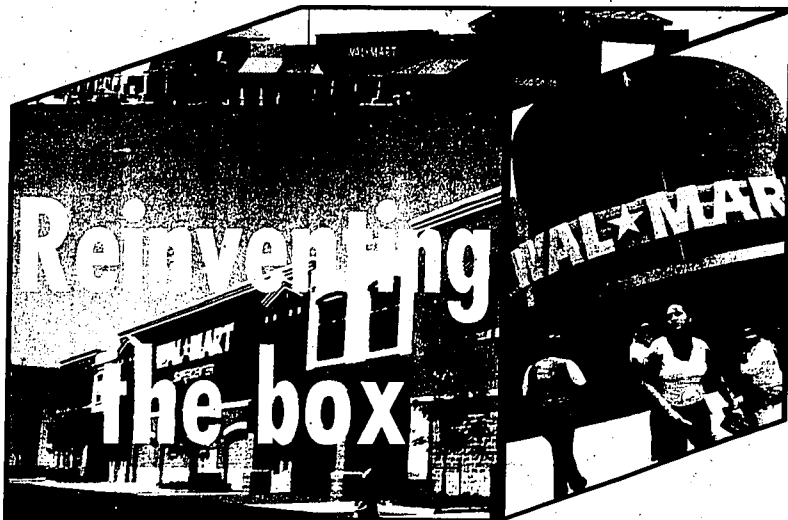
Photos show three different Super Wal-Mart stores with different designs. Wal-Mart, faced with controversy when it moves into new towns, created a new prototype that features a broken plane — different levels of roof tops — enabling it to be more easily customized to different communities.
