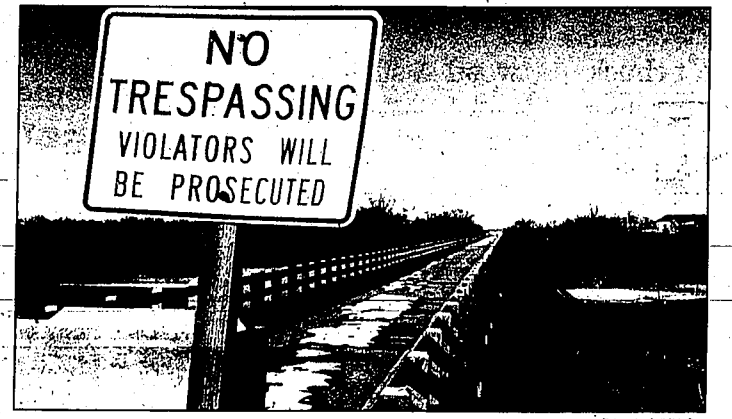
Despite rotting and bulging wooden pilings, a group of Mini-Cassia residents are trying to save Jackson Bridge at 200 N. 800 E. in Mindolota County.
