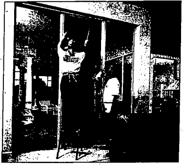
Lightly tinted window film being professionally installed on a sliding glass door. Large glass areas are more difficult to do yourself.
