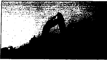
The sun sets behind a bulldozer used for the demolition of houses in the Jewish settlement of Peat Sadeh on Sunday in the Gaza Strip.
