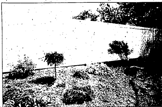
This is a view of privacy fencing with a decorative lattice top and standard post caps. Even with the lattice top, it still blocks the direct force of the wind.
