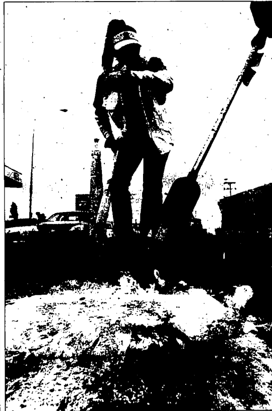
Stacy DeRuiter of Road Work Ahead of Twin Falls removes thermal plastic from a crosswalk Wednesday afternoon on Blue Lakes Boulevard North while Ed Martin melts the plastic with a torch. The crew will continue re-stripping the four crosswalks today, and various lanes will be closed periodically.
