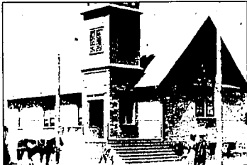
The Living Waters Christian Community church at 262 Fifth Ave. E. in Twin Falls. The church originally was the Twin Falls First Baptist Church, built between 1905 and 1908.
