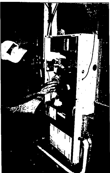
Older gas furnaces allow for a little more home maintenance than newer condensing furnaces.
