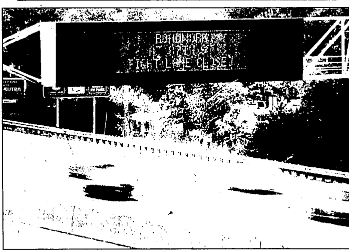
An electronic sign at I-35 and Johnson Drive in Shawnee, Kan., alerts motorists to traffic problems ahead. The sign is part of the KC Scott system that uses cameras and road sensors to monitor traffic. Missouri is looking into a state-wide cell phone system to do the same thing.
