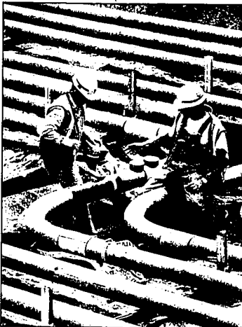
Workers are shown among pipes at a waste treatment plant being built at the Hanford nuclear reservation near Richland, Wash., in this 2004 file photo. The plant could cost billions of dollars more than first estimated and take an additional four years, a newspaper reported on Thursday.
