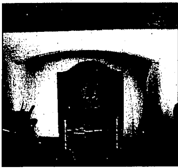
Decorative cast iron fireback is placed in the rear of an open fireplace to radiate more heat out into the room.
