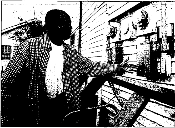
Walter Vine, an experienced contractor, used his knowledge to cut through the red tape to get power to his home and others on his street who have returned home. Vine said his uncle a licensed electrician certified the work.
