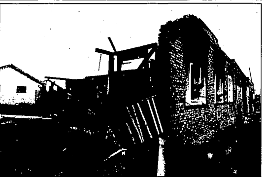
The charred shell of a city-owned warehouse is all that remains Friday afternoon following a Thursday night fire near Railroad Street and Maxwell Avenue. The building, owned by Twin Falls Urban Renewal Agency, was empty at the time of the fire.
