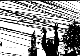
A Baghdad resident inspects wires that connect houses to private generators Sunday in Baghdad. The capital's power supply has worsened since the 2003 overthrow of Saddam Hussein despite billions of dollars set aside by the Bush administration for reconstruction.
