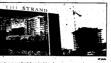
New luxury condominiums and townhomes are seen under construction Thursday in Portland, Ore. New economic data shows that construction fell in all regions of the country except the West, which saw an increase of 7.9 percent last month.
