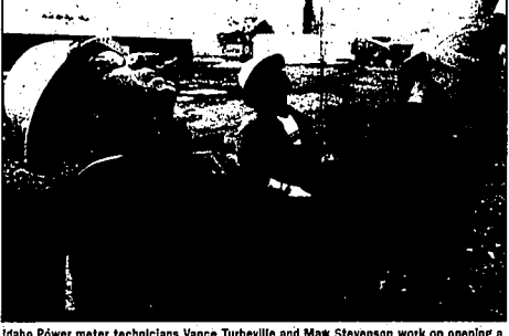
Idaho Power meter technicians Vance Turbeville and Mark Stevenson work on opening a transformer fuse Sunday near Ross Street North In-Twin-Falls.
