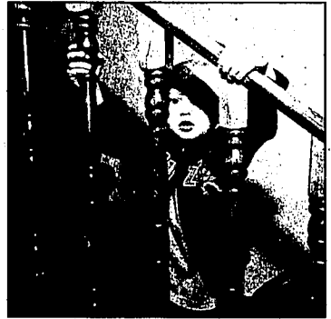
Three-year-old Caleb Bonnes peeks through the balusters of the stair railing in his Twin Falls home. The Bonneses added additional balusters to reduce the chance of a child getting stuck in or falling through a wide gap. The Bonnes home was built in the early 1980s, when the code did not require a smaller gap in stairway railings as it does today.
