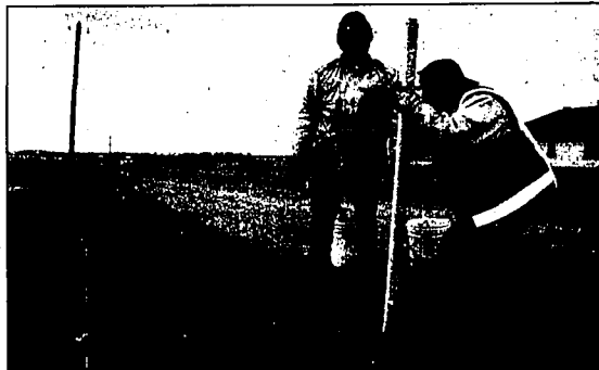
Javier Leija, right, and Arturo Triana, both of Idaho Sand and Gravel of Jerome, work on Washington Street South. The half-mile stretch of road leading to Joslin Field, Magic Valley Regional Airport, is closed, and drivers must take a two-mile detour.
