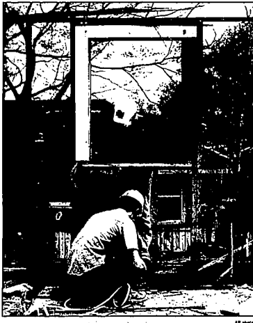
Asher Griffith top, and Jeremy Maxwell-Parish salvage what they can from a home damaged by Hurricane Katrina in the Lower Ninth Ward of New Orleans last month. Wood and other materials they salvage will be re-sold at the Green Project, a nonprofit recycling center.
