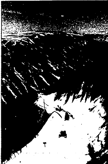
Three snowblowers work their way through a 7-foot-deep drift Friday, just above Vista Point on the Beartooth Highway near Red Lodge, Mont. The lead plow has a 7-foot-tall-by-8-foot-wide blower that will kick out rocks up to 8 inches in diameter. The chains for each tire of the plow weigh 575 pounds. A media campaign is planned as a way to publicize the Beartooth Highway's readiness for traffic this summer, after a 2005 closure that hurt commerce in Red Lodge. The owners of Herring Cycle and Ski shop said the highway's closure triggered by rock and mud slides, followed by a $14 million repair project, reduced their business by 30 to 40 percent.
