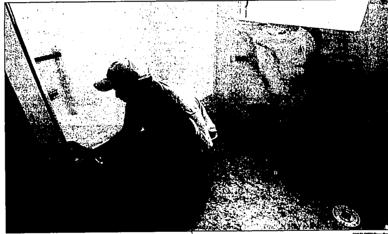
Forrest LeBaron, of Forrest LeBaron Drywall Inc. of Twin Falls, brushes down a wall at the Habitat for Humanity home in Buhl. The drywall company was one of many businesses that donated materials and labor to help build the home.
