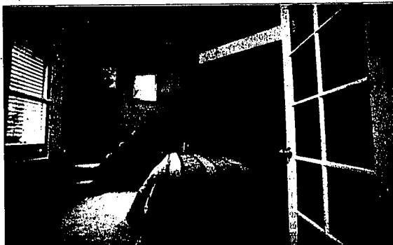
The Beltrons had difficulty attaching French doors leading to the master bedroom because of two-foot-thick walls, made of stone.
