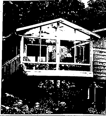
This patio room has sliding windows throughout for 50 percent open screen area. Notice the ceiling fan for evening when the breezes die down.
