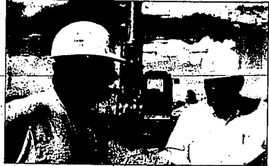
Roger Alford, left, of Strzkan Excavating, discusses the damage to his backhoe with Leonard Bay, project supervisor with STARR Corporation, Monday afternoon at the new school site in Jerome.
