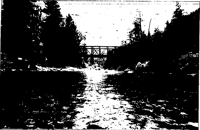
A bridge for the Virginia Gulch trail spans the South Fork.
