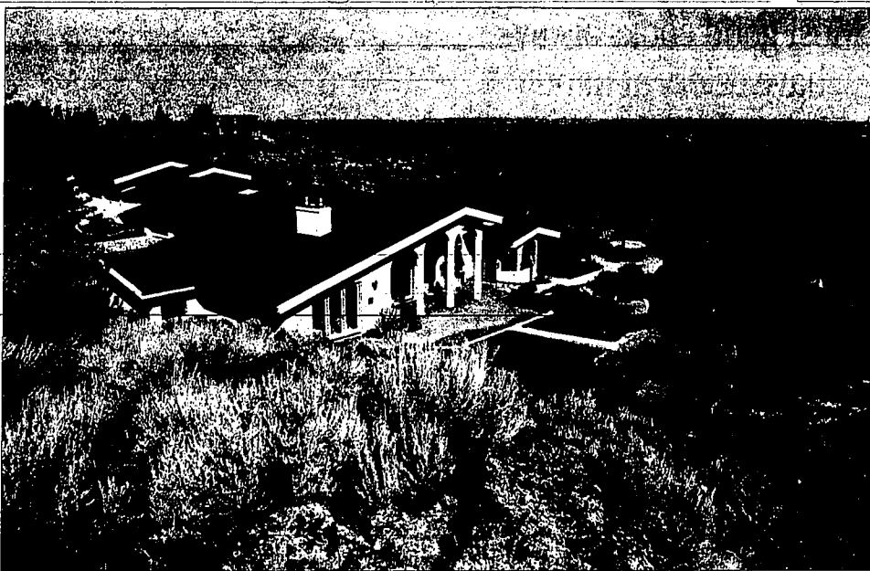
Janet and the late Charles Wojcik built this 5,500-square-foot home along the canyon rim near Kimberly more than 12 years ago. The couple spent $250,000 on a road to access the site and on chipping away the rock.
