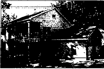
This house has a steel frame made of a combination of galvanized and red iron framing members. The exterior is finished with brick.
