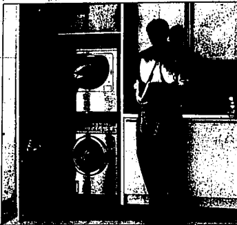
A European-style front-loading washer and dryer are located in a closet. Condensing clothes dryers do not require outdoor venting.
