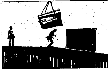
Workers build a cover for a clarifier recently at the Coeur d'Alene Wastewater Treatment Plant in Coeur d'Alene.
