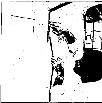
Replaceable vinyl weatherstripping seals well on the hinge side of the door because it gets compressed with little rubbing and wear.
