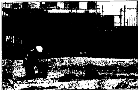
The work must go on even in a snowstorm. Jason Sollars of Alet's Electric Inc. prepares the ground Monday morning in Jerome at the site of the new elementary school to install a transformer. Today's forecast for the Magic Valley calls for a chance of snow with a high of 25.
