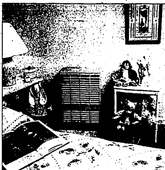
This small direct-vent gas heater uses no electricity. It produces about 10,000 Btu/h, enough to heat a small to medium-size room.
