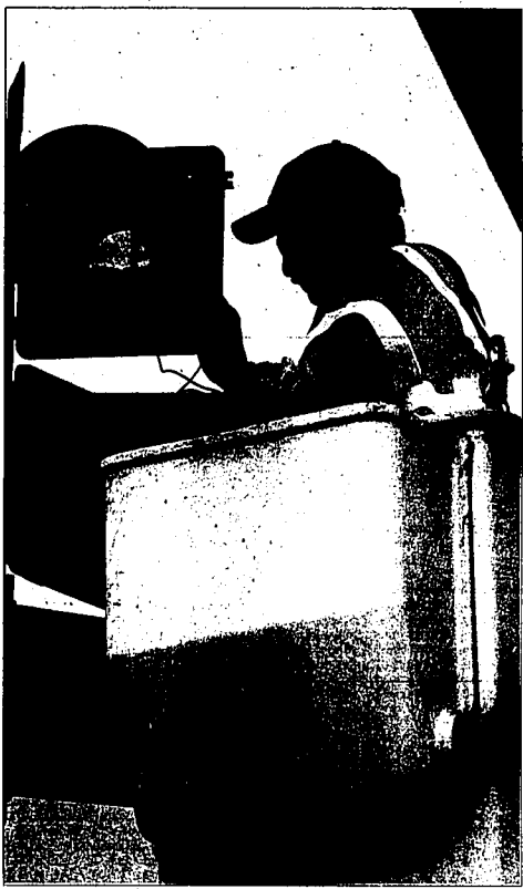
Jon Leazer, a journeyman electrician with the city of Twin Falls, changes the bulbs in a traffic light Thursday at the corner of Hayburn Street and Blue Lakes Boulevard North.
