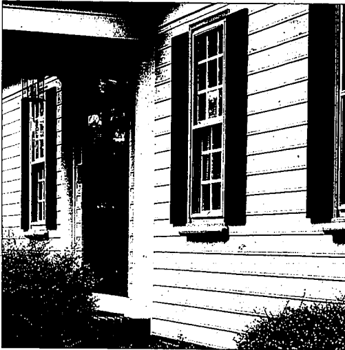
Fiber-cement siding is durable and relatively lightweight and simulates standard cedar lap siding.
