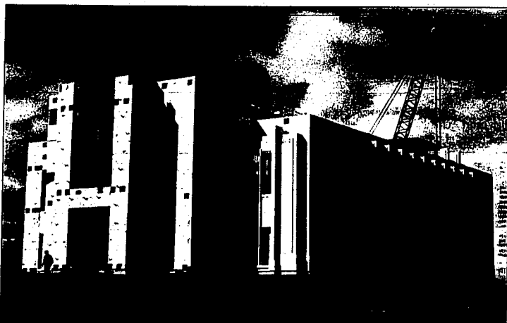
Pre-cast cladding panels were applied Monday to The Church of Jesus Christ of Latter-day Saints temple along Eastland Drive in Twin Falls.
