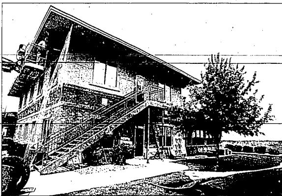
Steve Gordon of Could Nine Construction puts up netting Wednesday at the Western Real Estate Group building, 139 River Vista Place. Workers have already installed the netting at the neighboring Premier Insurance building in an attempt to stymie the thousands of cliff swallows that have nested at the building in each of the past two years.
