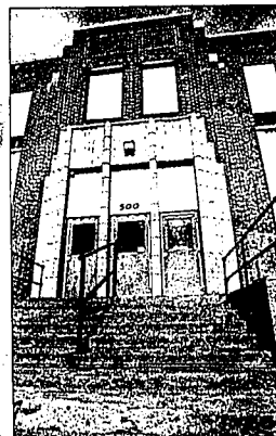
The Washington School building was built in 1931 and was owned by the Jerome School District until May 18, when Magic Valley Christian School purchased the building.
