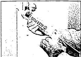
Siliconized acrylic latex caulk can be used for most outdoor and indoor caulking jobs. It cleans up with just soap and water. Photo courtesy of DAP
