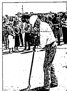
Gov. Butch Otter ditched his jacket, put on a hard hat and grabbed a shovel Friday to dig the first shovelful of dirt at the groundbreaking for the new Con Paulos car dealership in Jerome.
