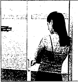
This retractable screen door on a sliding glass patio door uses magnetic latches to keep it in the closed position and retracts into a small roll on the side of the door when open.
