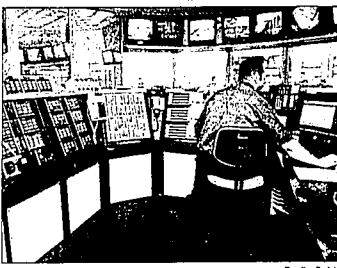
Twin Falls County Sheriff's Department Deputy Terry Hawkins runs the switchboard at the Twin Falls County Jail in June 2006. The jail's main control board, which controls the intercom system, TV feeds and door locks, is outdated and will be replaced with a new digital board.
