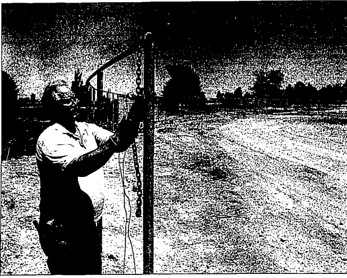
Marc James, construction supervisor for the College of Southern Idaho, installs the outfield fence around the college's future softball field. CSI officials say the team may have to wait to play on the field because the outfield grass needs time to take root.
