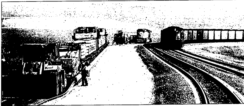
A section of triple-track rail is put in place last month south of Gillette, Wyo., where BNSF Railway is adding to its rail network in Wyoming's coal producing region, the Powder River Basin.
