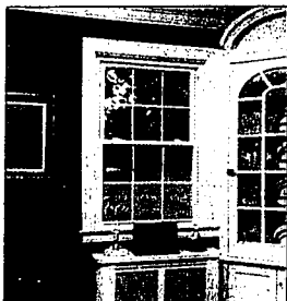
This vinyl double-hung window has simulated divided lites and insulating foam injected into the cavities in the frame.
