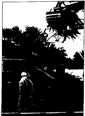
Workers with the United Rebuilder Group demolish a home in Chalmette, La., July 11. Contractors hired to clean up after Hurricane Katrina are fuming over delays in getting paid by FEMA, and some fear the red tape will discourage companies from bidding on the big rebuilding projects that lie ahead for New Orleans.
