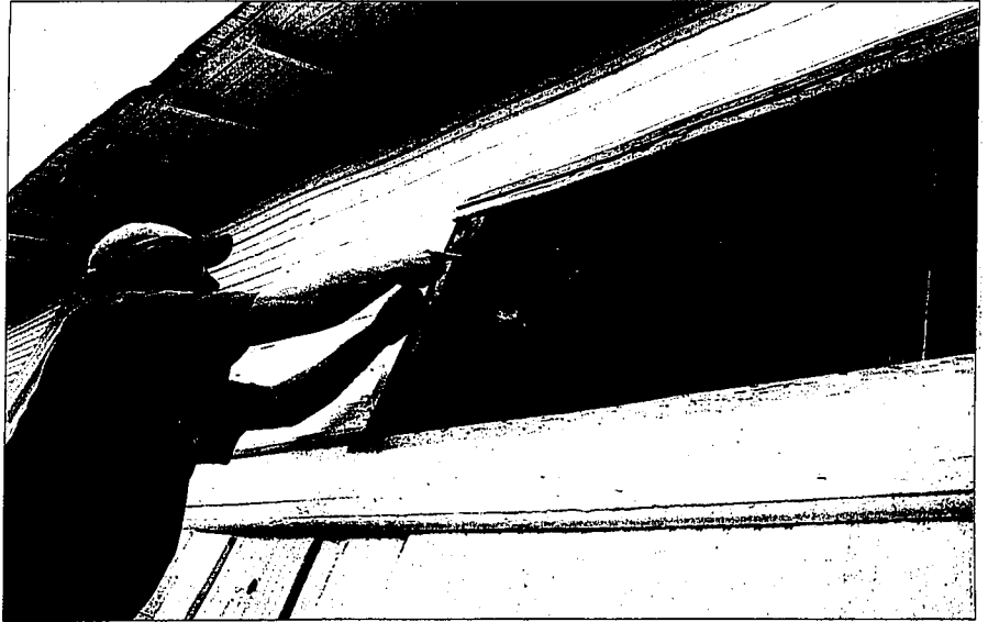
Chad Scovel, left, and Daniel Paz work on replacing a window Monday morning in Twin Falls. Paint Magic's current project is the house of Rosemarie Denning of Twin Falls.
