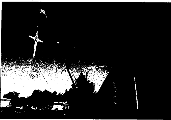
A crew from Stutzman Inc., positions a new cross Friday morning on the pitch of Immanuel Lutheran Church in Twin Falls.
