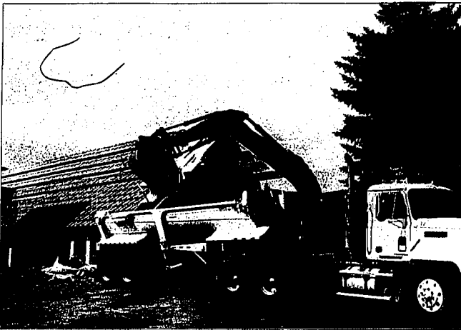
Brently Whitsett of Belleuve operates a Caterpillar lifting pieces of Our Lady of the Snows Catholic Church into a waiting Erwin Excavation truck in Sun Valley earlier this week.
